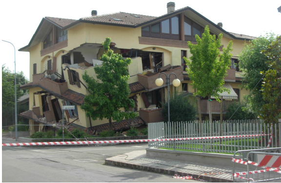
Figure 1. Example of damage to a building due to the Emilia earthquake in 2012.
